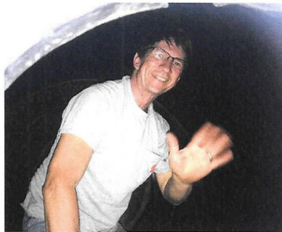
Paul kneeling inside an FOH water tank as assembly begins
